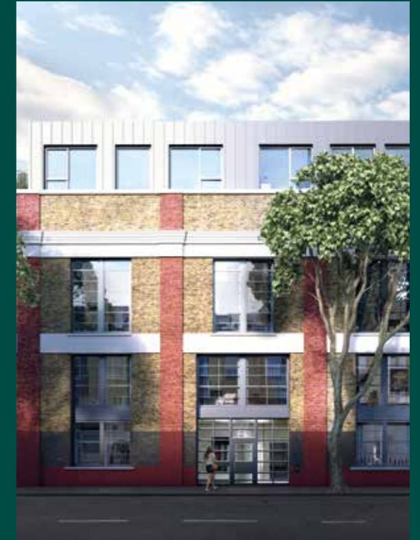
Arlington Lofts, Camden
